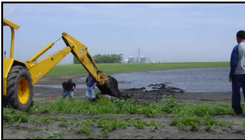
Breaking drainage tile for a wetland restoration in Hawk Creek Watershed
