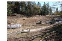
Reshape the gully head
