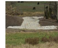
Construct a rock-lined waterway
