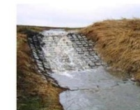
Build a grade stabilization structure
