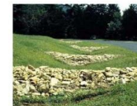
Install grade check dams
