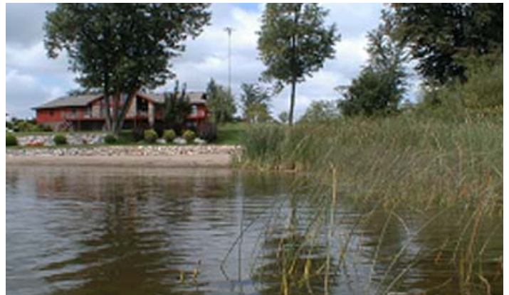
The vegetation on the right reduces the energy of waves, which is a natural solution that does not carry the cost or impact of riprap seen on the left.
