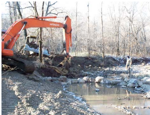
As part of the new watershed project, work began in December of 2002 to help stabilize 1,000 feet of eroding stream bank in Seven Mile Creek Park. The project demonstrated alternative techniques to slow bank erosion while at the same time helping increase habitat for brown trout.
