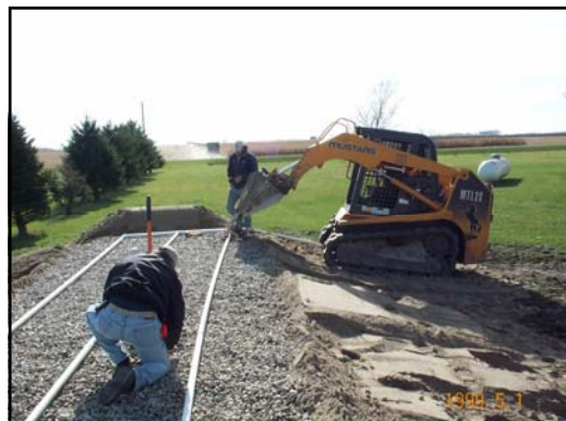
33 septic system were upgraded from 2002-2004.
