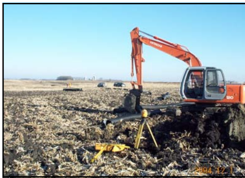
Modifying Public Tile to be routed through a recently restored wetland for water quality, flood reduction and habitat.
