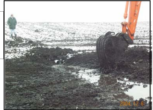
Creating outlet ditch for private tile to be routed into wetland.
