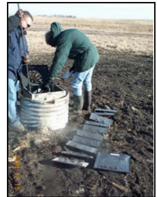
Installing drop logs in the water level control structure.
