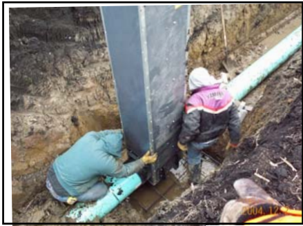
Connecting the in-line water level control structure
