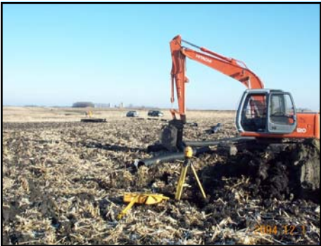
Locating county main to be modified for drainage into wetland.
