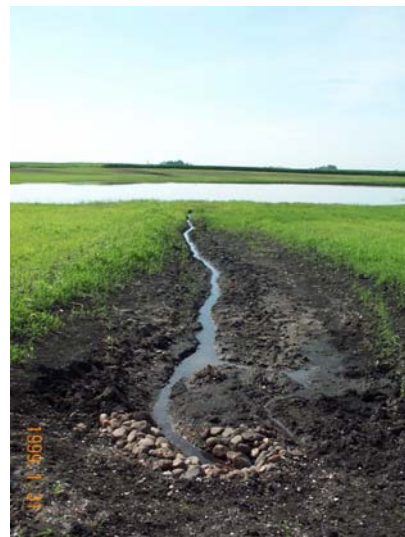
Adjacent drainage tile routed into newly restored wetland basin
