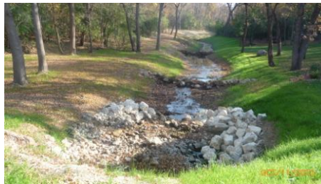
City of Savage Utica Ravine Project (before and after) reduced sediment to the Credit River by 50 tons per year
