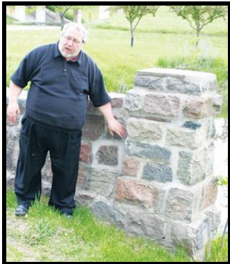
City manager Steve Jones points out where a crack has opened in the wall of one of the historic WPA stone bridges in Lagoon Park. City Council members toured the park at the end of June to view damage by spring floods.
