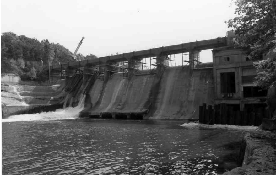
The Rapidan Dam on October 8, 1983 (upstream, during rehabilitation)
