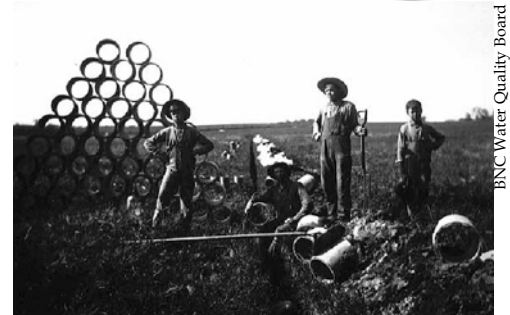
In the beginning tiling was mostly done by hand using a spade to lay concrete or clay tile.
