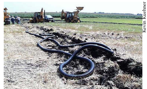
Modern corrugated plastic drainage tile
