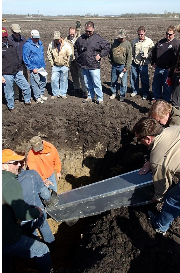
A water-control device is hooked to a field drainage tile on Don Wenner's farm land near St. Peter. The control structure, which can hold back some water and nitrogen in fields, is the first in the state to be used in a field. It's effectiveness will be tested by researchers from several agencies and organizations. John Cross / The Free Press
